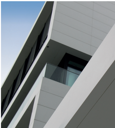
Microsoft Germany Headquarters, Munich, DE © Andreas Frisch, GSP Architekten
