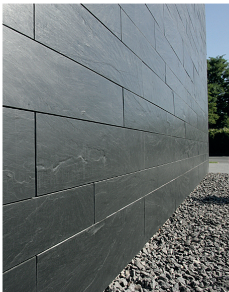
Rathscheck office and training building, Mayen, DE © Rathscheck Schiefer
